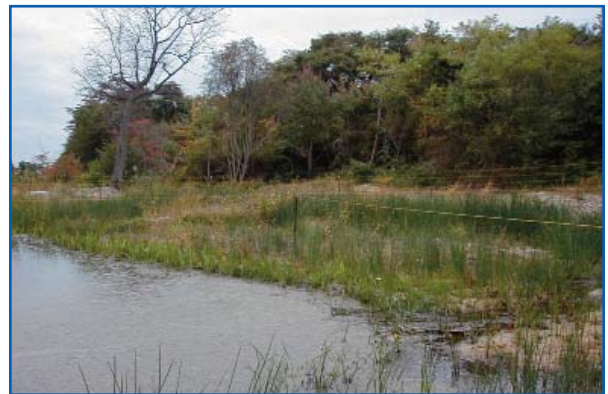
A constructed wetland system on Ketcham's Creek helps remove nonpoint source pollution from stormwater runoff.
